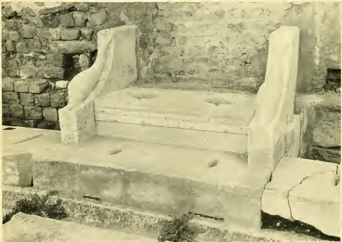
Fig. 12. A LATRINE near the Forum of Tingad in Algeria, flushed with water from a constant fountain
